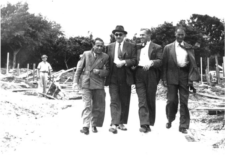
Fig. 2.2 Weizmann, with Arieh Elhanani and Israel Dicker, the Institute architects, in the building site (1947). Courtesy of Nima Geffen
