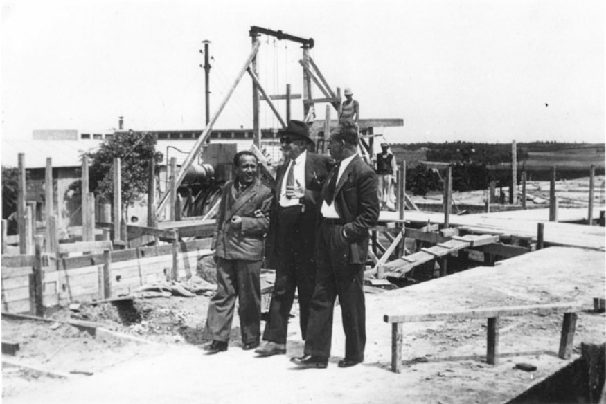
Fig. 2.3 Weizmann, with Arieh Elhanani and Israel Dicker, the Institute architects, in the building site (1947). Courtesy of Nima Geffen
